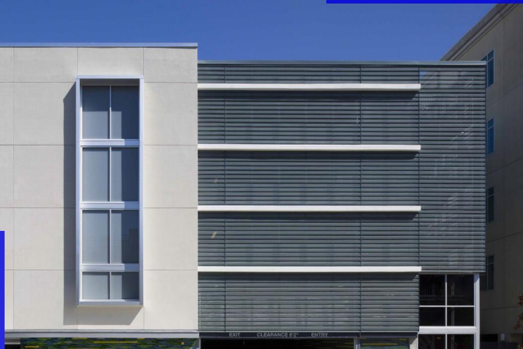
Carefully configured on a tight site, this 88,500 SF concrete structure includes 230 spaces on six-stories above-grade and one level below-grade that connects to an adjacent underground garage of a medical office building next door.
